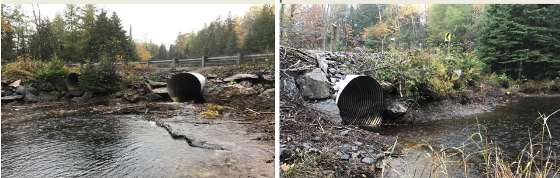
Figure 25 Eel's Lake Road Culvert (BCI=56 Fair)
