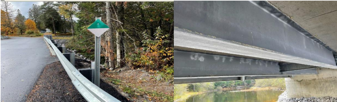
Figure 23 Tall Pines Bridge (BCI=52 Fair )
