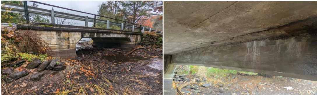
Figure 24 Universal Road Twin Culvert (BCI=82 Very Good)
