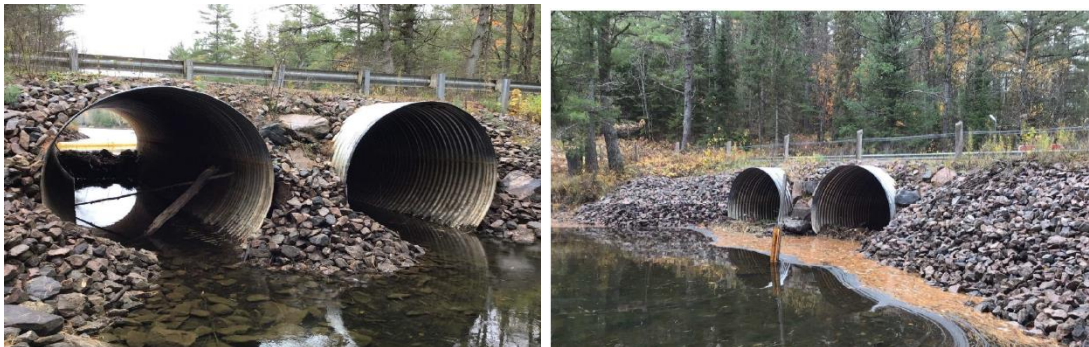
Figure 24 Universal Road Twin Culvert (BCI=82 Very Good)
